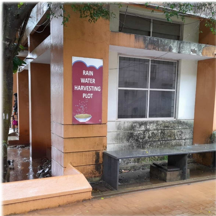
Rainwater harvesting plot
