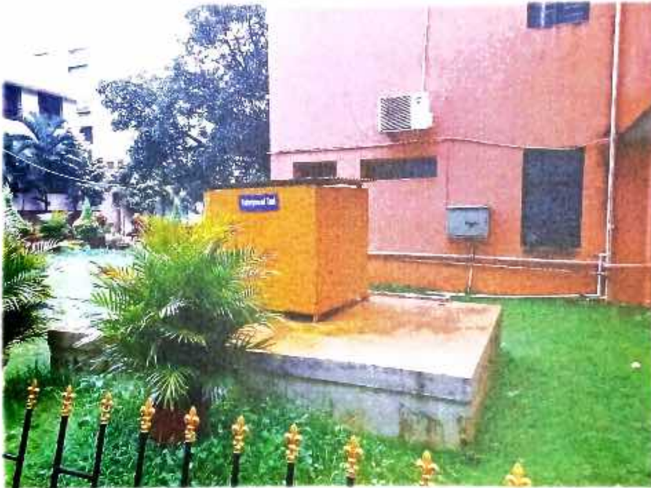
Underground water tank
